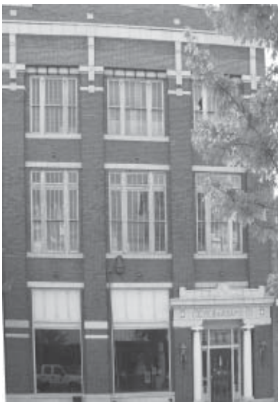
Geyer & Adams Building
